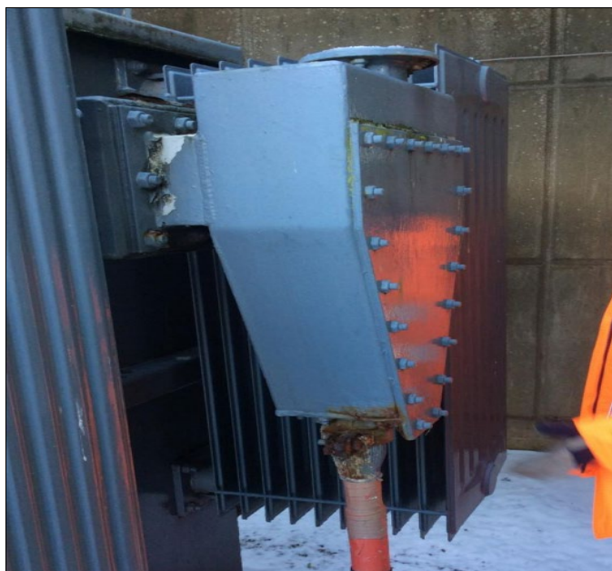
Figure 5: Corrosion on the radiator fins and connecting cables
