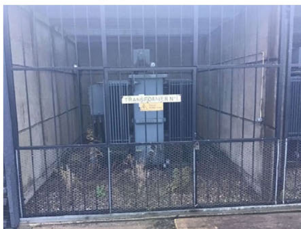
Figure 4: Plant 1 T1 Transformer 1 currently isolated
