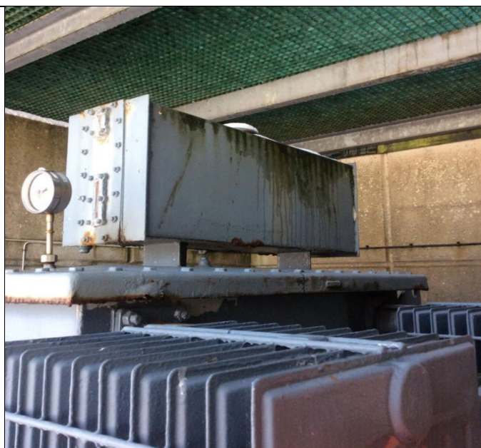
Figure 6: Leaking oil from conservator tank and corrosion
